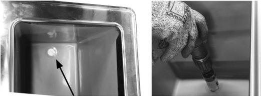
C. Apply thin ring of plumbers putty around the drain.
