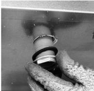
F. Tighten the nut with channel locks, use a fork to hold the drain in place if necessary.
