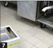
Position SDU under drain extension.
