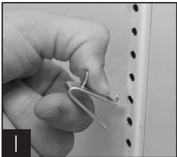
1 Installing top tab of shelf clip
