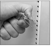
Fig. 6. Installing top tab of shelf clip.
